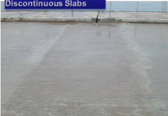
Strengthening by Joining Discontinuous Slabs
