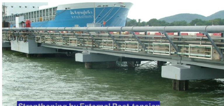
Strengthening by External Post-tension
