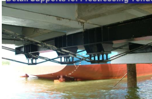
Detail Supports for Prestressing Tendon
